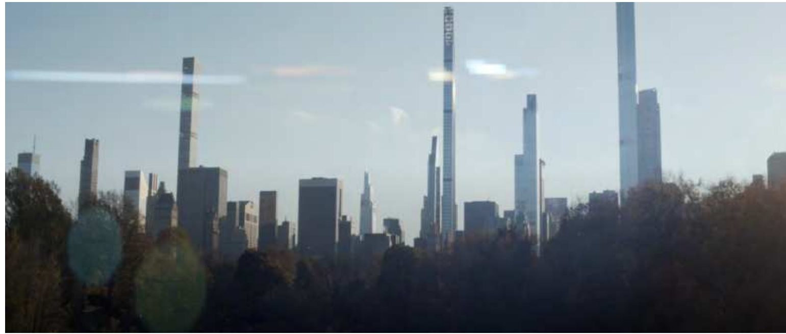
Manhattan's Billionaires' Row, looking south from Central Park, with the new generation of pencil towers, a design inspiration for their level of luxury and sky-piercing purpose
